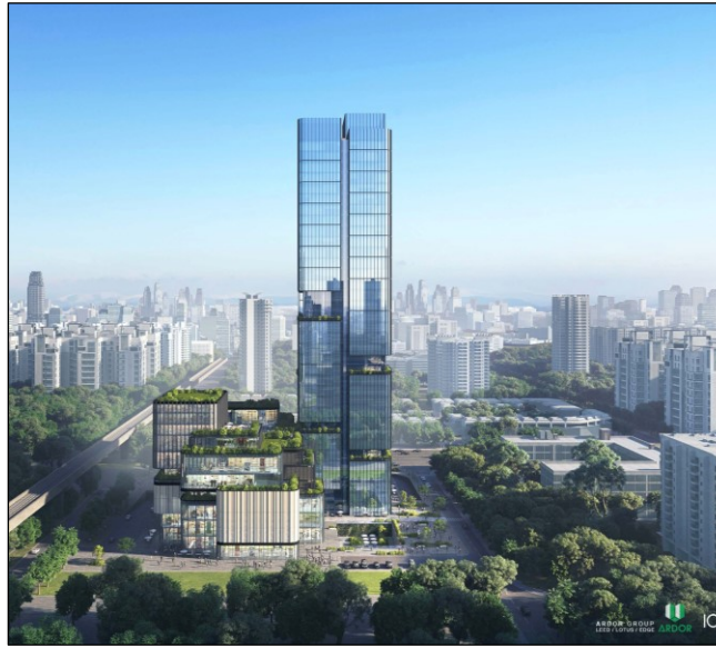
Starlake Urban Complex, LEED Silver
